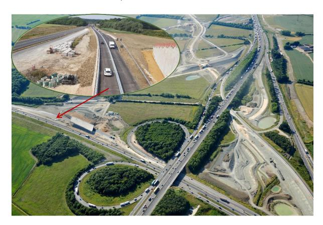
Along the Cambridge Northern Bypass, the lengthy period of night work required for phase 1 of the work will soon come to an end. During this time we have removed the safety barrier from the centre of the road and resurfaced it so we can move traffic over to construct the widened section of this part of the A14. During phase 2 the majority of the work will be carried out during the day.
